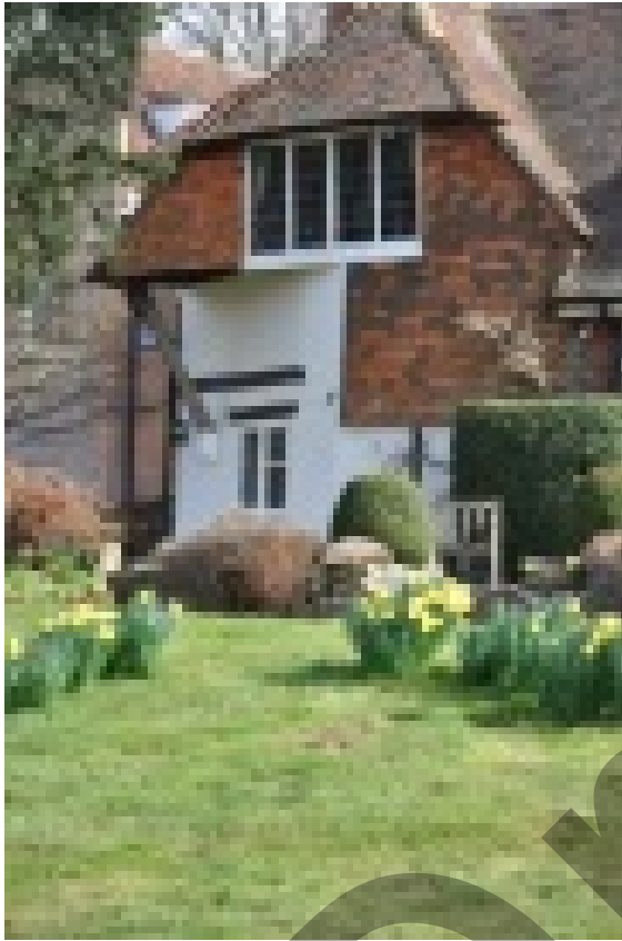
Plain tile hanging and painted brickwork
