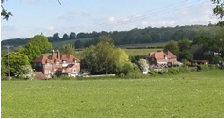
Former Brickyard Cottages (rear)
