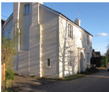
Former Moor Hall lodge
