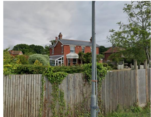
Figure 18. View northeast to Grantham House
