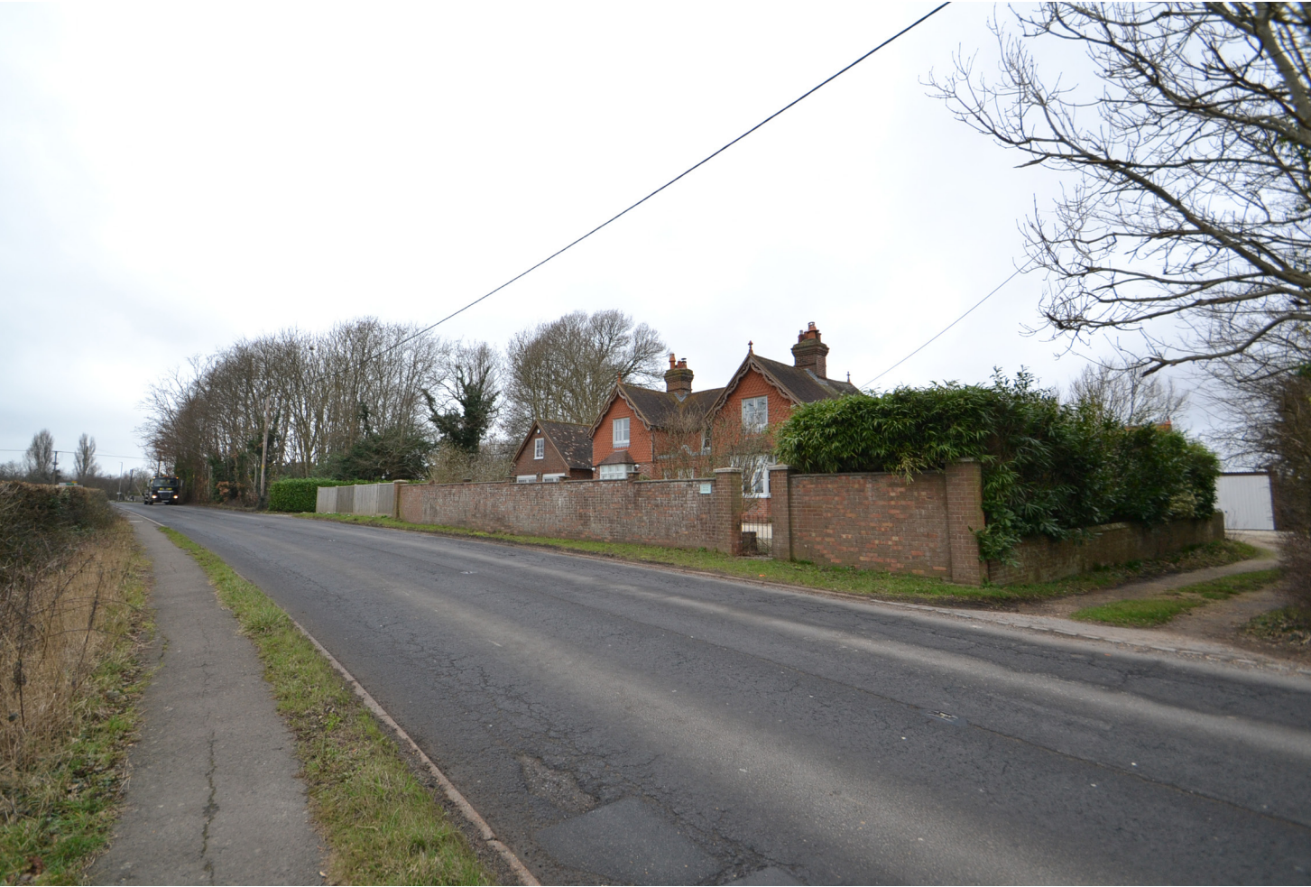
Plate 1 View of Brook House from A271, from where the architectural interest of its principal elevation can be understood and appreciated
